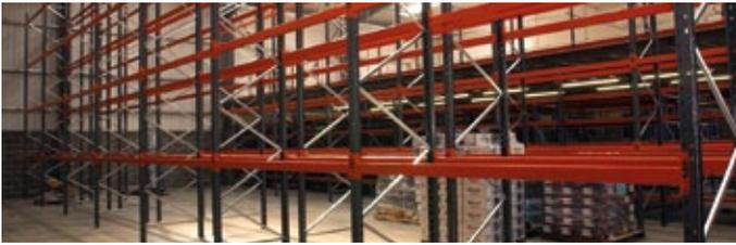
South Wales based retailer Peacocks has a major distribution centre in Treforest and Albion Workplace Solutions has recently installed a major shelving installation on a mezzanine third floor, fitted three tiers high (29 lanes of 6 bays).
